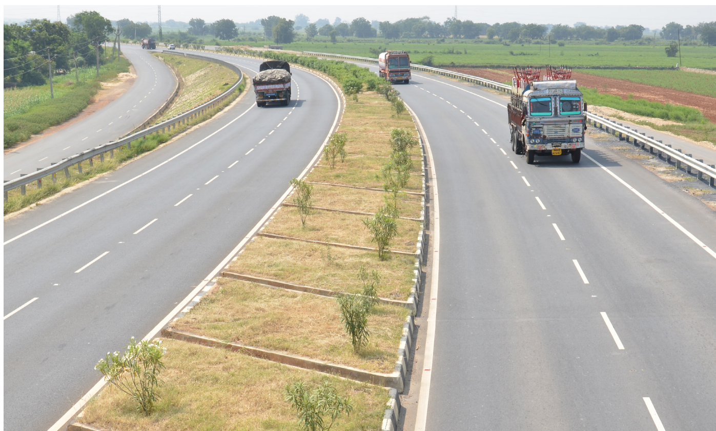
Kadapa-Kurnool Section of NH-40, Andhra Pradesh
