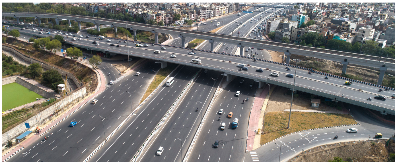
Interchange at Akshardham Junction, Delhi-Meerut Expressway, Delhi
