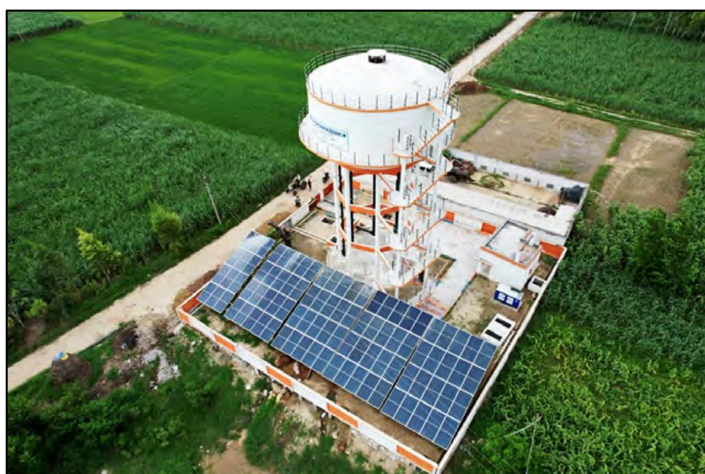
Water Supply Scheme in Muzaffarnagar, Uttar Pradesh
