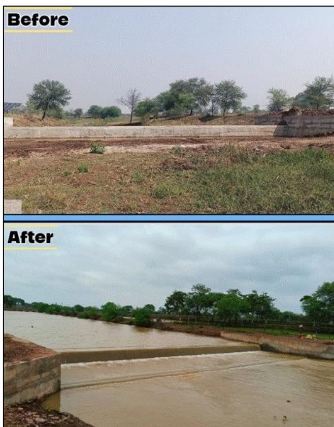
Check Dam in Balod District, Chhattisgarh
