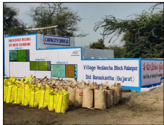
Image 3: Greywater Treatment Plant in Vedancha
