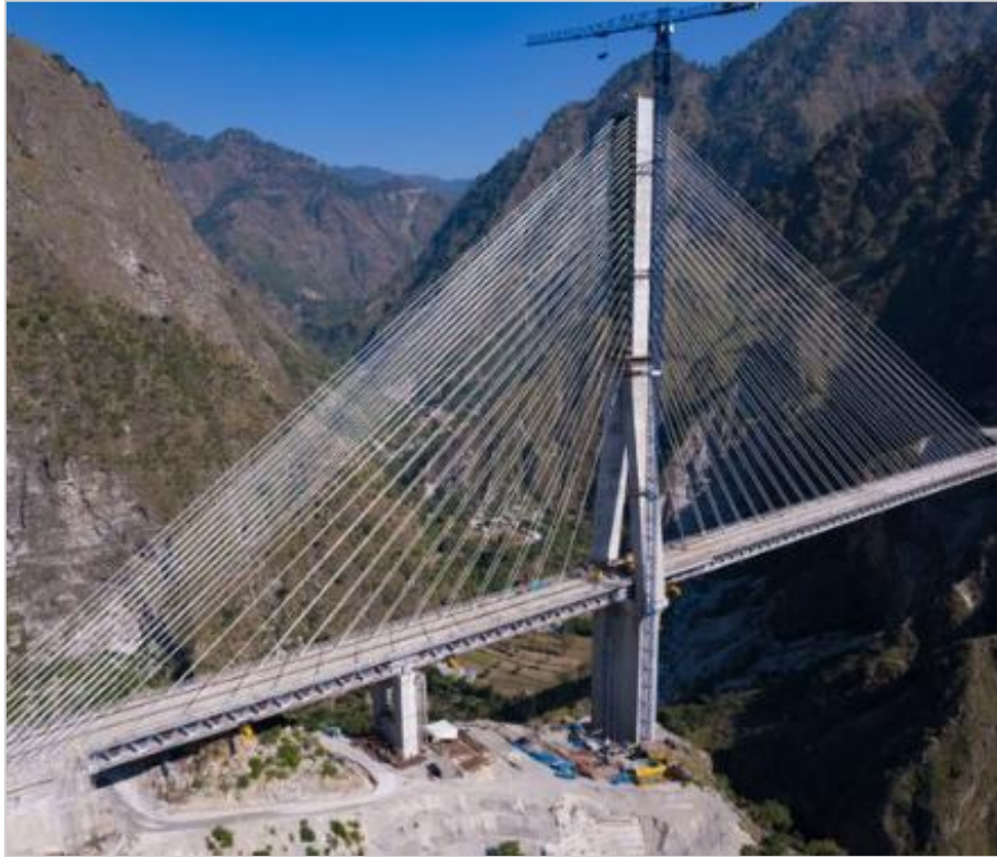
Image 3: Anji Khad Bridge in Jammu and Kashmir
