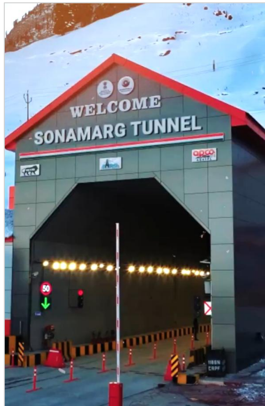
Image 5: Sonamarg Tunnel, Jammu and Kashmir
