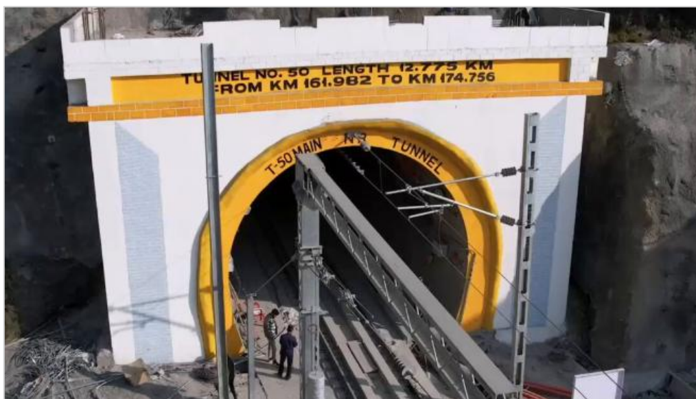
Image 4: Tunnel T50 in Jammu and Kashmir
