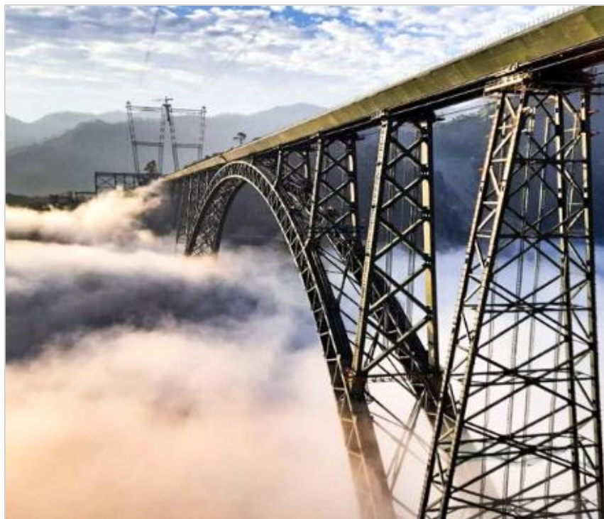
Image 2: Chenab Rail Bridge in Jammu and Kashmir
