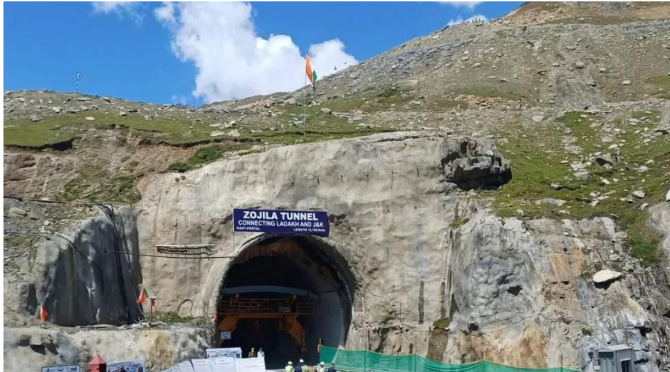
Image 6: Zojila Tunnel, Jammu and Kashmir
