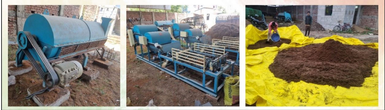
Coconut Waste Processing Plant in Patna
