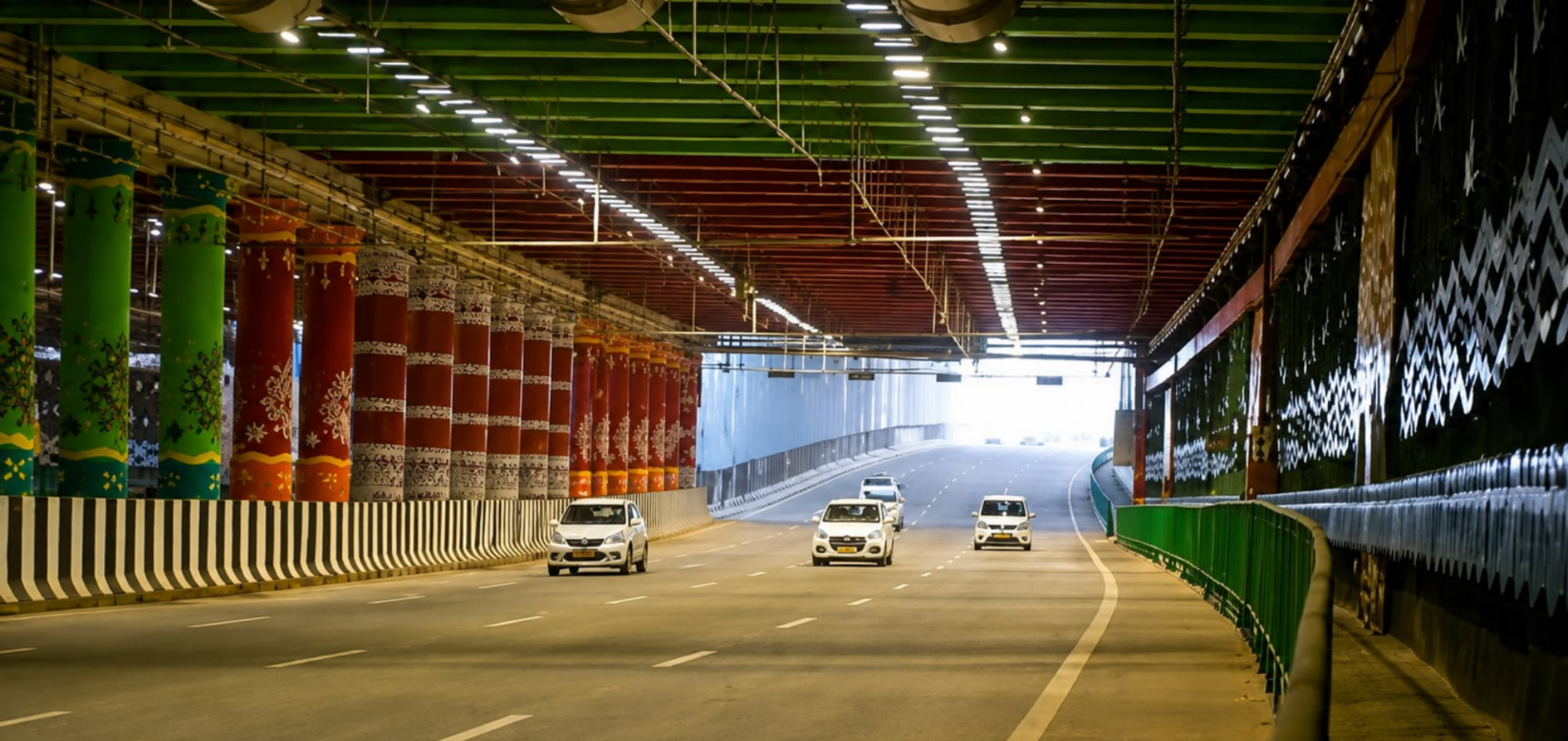
Construction of Six-lane Dwarka tunnel in Delhi (8 km; Rs 6,970 Cr)
