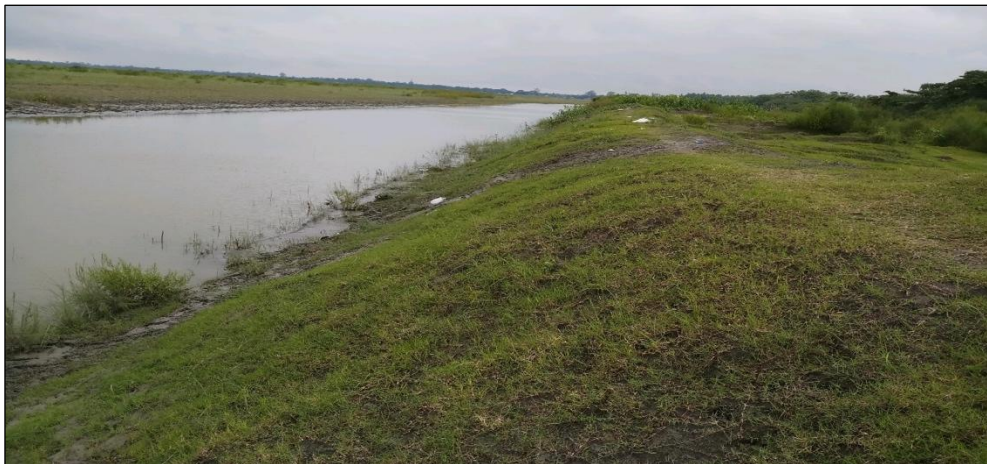
Post construction of Bank revetment work at Sumoimari, Majuli, Assam.
