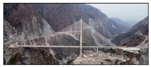
About 80 kilometres from Jammu city, the bridge is set against a striking backdrop of snowcovered peaks. Towering 331 metres above the riverbed and stretching 725 metres across, it is anchored by 96 high tensile cables. At its heart stands an inverted Y shaped pylon that climbs 193 metres above its foundation. The total length of cable strand used in the bridge is an impressive 653 kilometres. Remarkably, the entire structure was completed in just 11 months.
