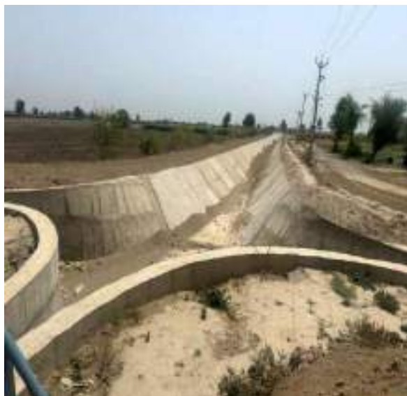
Cement Concrete Lining of Bahadurke Distribution System of Jalalabad Branch
