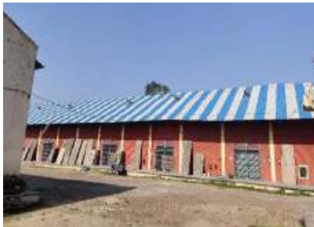
Replacement of old Asbestos Sheet Roofing of godowns with Galvanized Iron profile sheet
