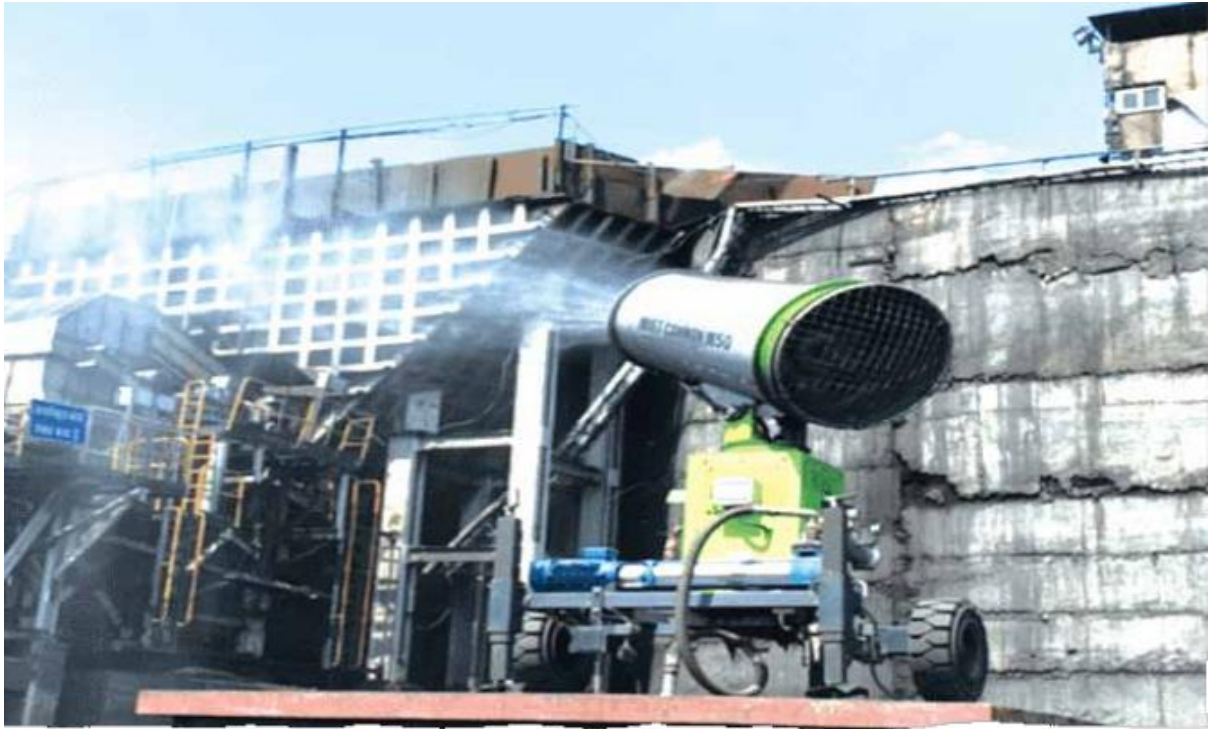
Fig. Mist Gun operation to control dust
