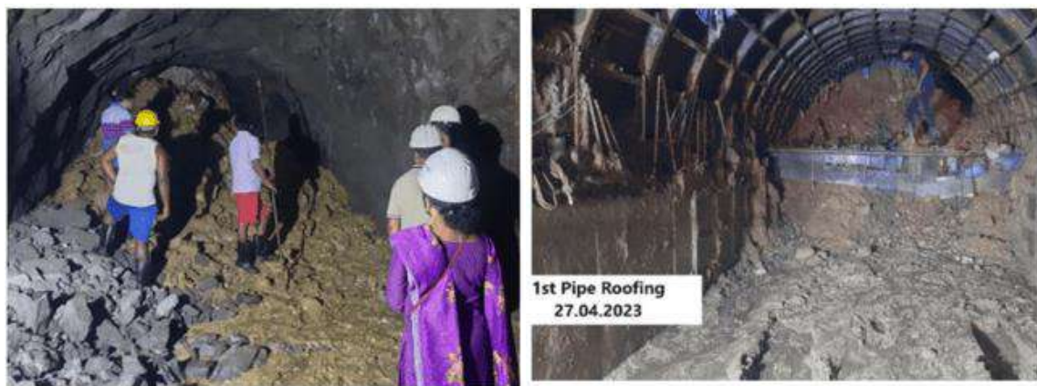
Plate 1: 1 st Collapse from face-IV, ingress of debris flow on 7 th January 2023 Plate 2: 1 st time pipe roofing was done on 27 th April 2023
