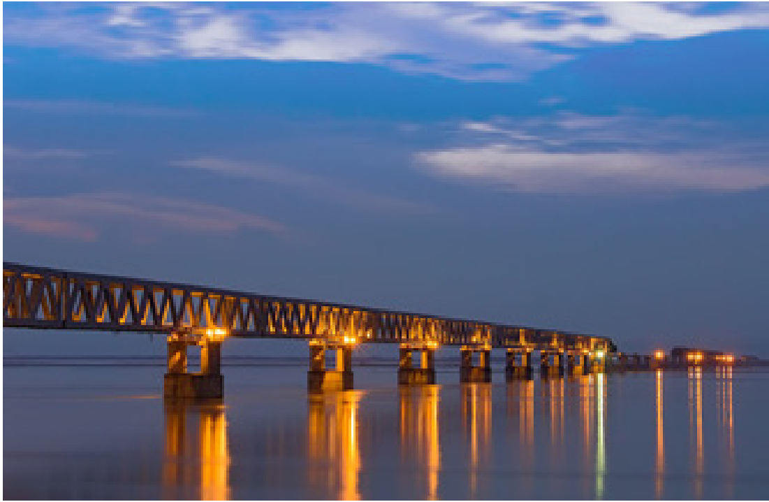
Bogeebil Rail-cum-Road Bridge
