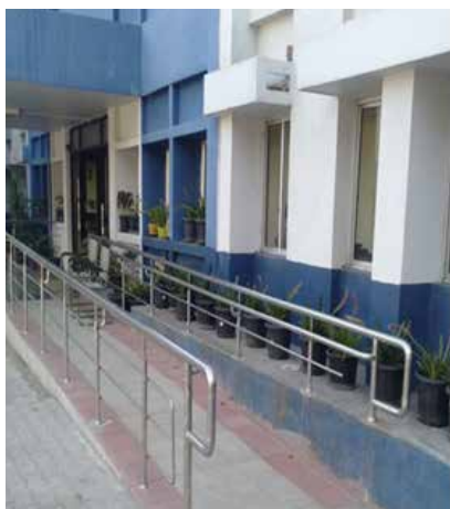
Ramp with double height handrails provided in Office of Accountant General, Kohima, Nagaland
