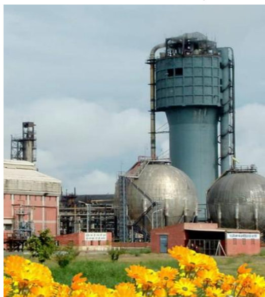
Green ammonia plant at Jubilant, Uttar Pradesh (Photo Credit: SAREP)
