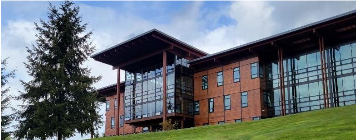
Tulalip Tribes Administrative Building modeled by WSU students for a renewable based microgrid feasibility study. (Photo Credit: Department of Energy)
