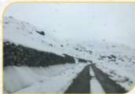
Thanguto Muguthang road in progress
