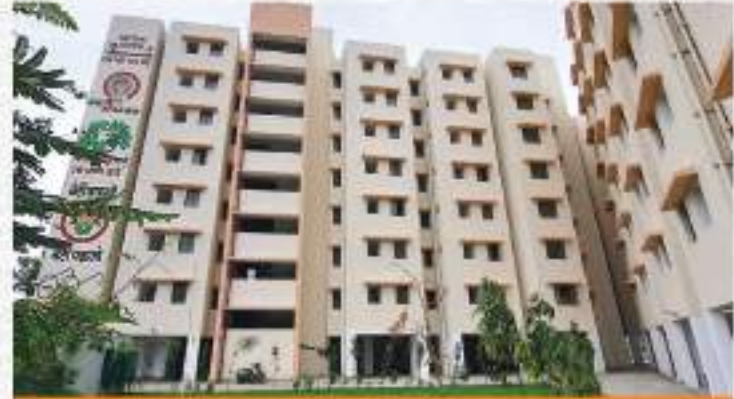
120 ISSR houses built at Bhudarpura in Ahmedabad, Gujarat
