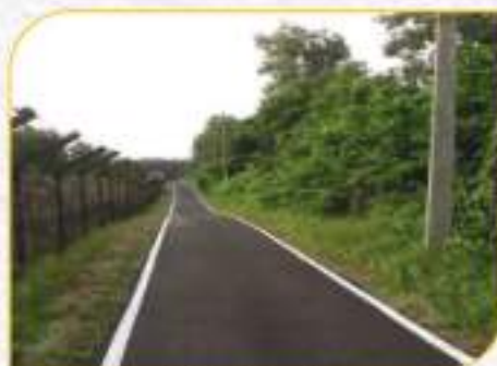
Repair of IBB Road in Tripura
