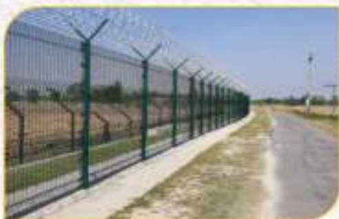
Replacement of border fencing in Siliguri Sector, West Bengal
