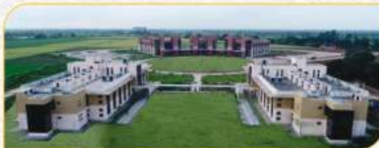
Administrative block, Library, Auditorium, School and Hostel building for ICAR- National Institute of Biotic Stress Management at Baronda, Raipur
