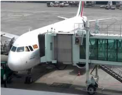
Aerobridges for obstruction free boarding in Chennai International Airport, Tamil Nadu
