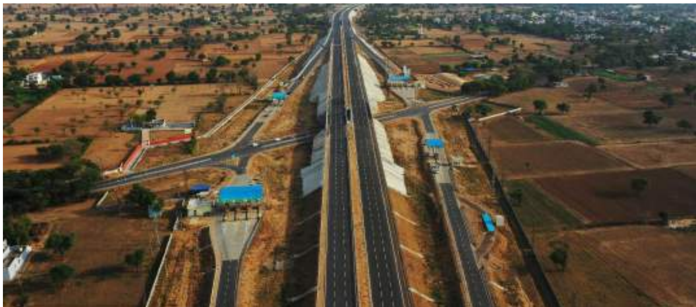
Interchange at Narnaul Bypass, Ambala – Kotputli Corridor
