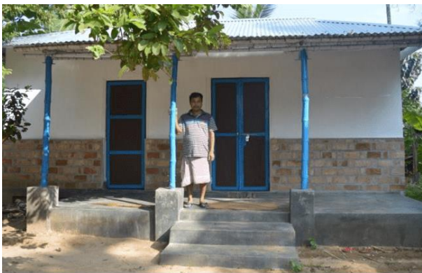
House with alternative construction technologies under PMAY-G in the State of Tripura
