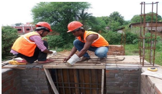
Placing of reinforcement steel
