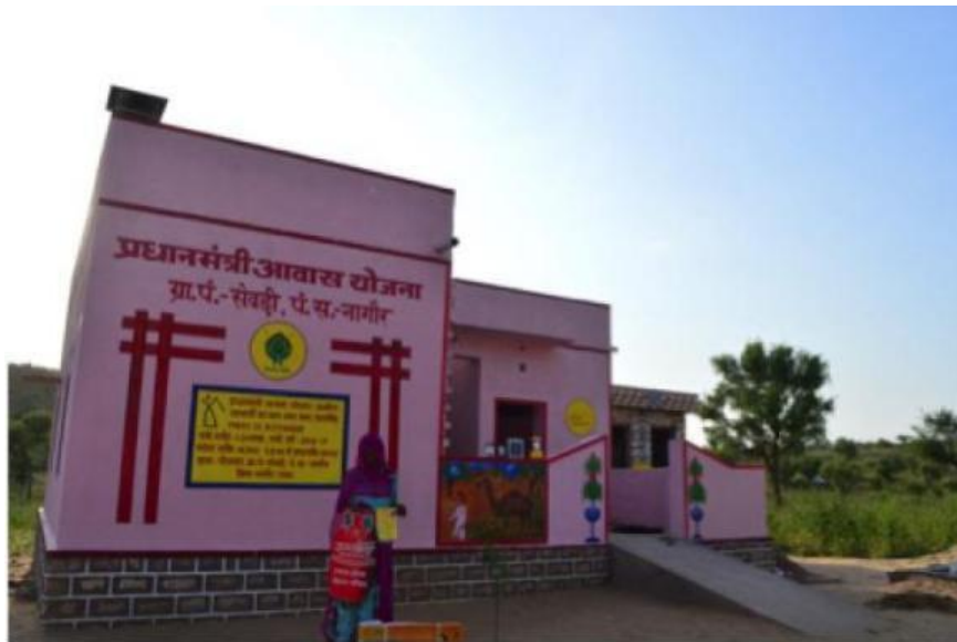
The home of Smt. Bhanwar Kanwar with Solar lights, LPG connection & toilet
