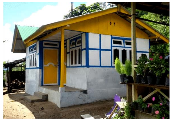
House with local construction technologies under PMAY-G in the State of Sikkim
