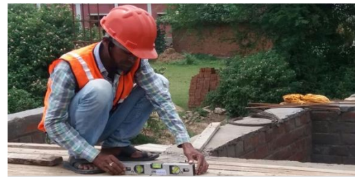
Leveling of Shuttering
