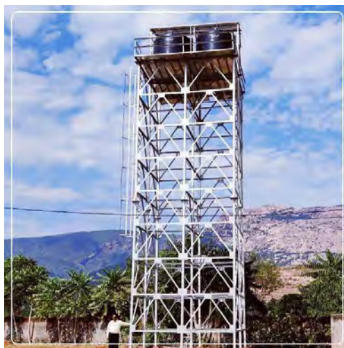
Overhead Tank, Chhattisgarh
