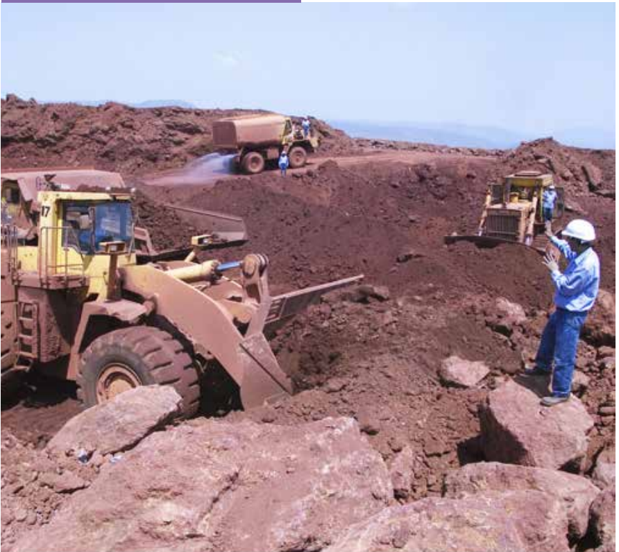
Mining Operation at Panchpatmali Bauxite Mines of National Aluminium Company Limited (NALCO)
